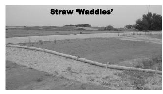
Ground covers can slow the flow of water reducing erosion and allowing sediment to settle out.
